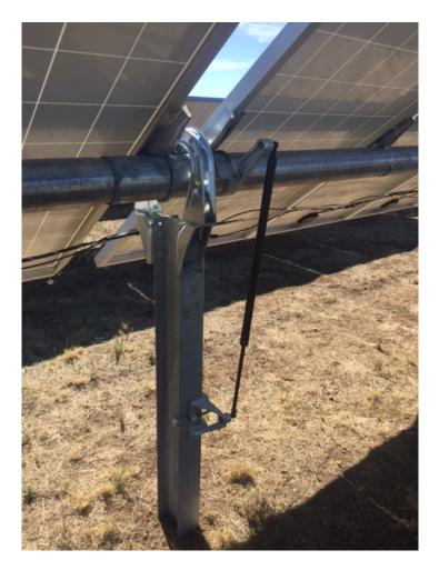
Intermediate support. The 5" EMT horizontal tube supports the panels. The rotation axis is above the tube. The columns are driven into the soil (30 seconds -typical drive time), using GPS to locate them. The brackets shown, allow slight adjustment, in 3 dimensions.
