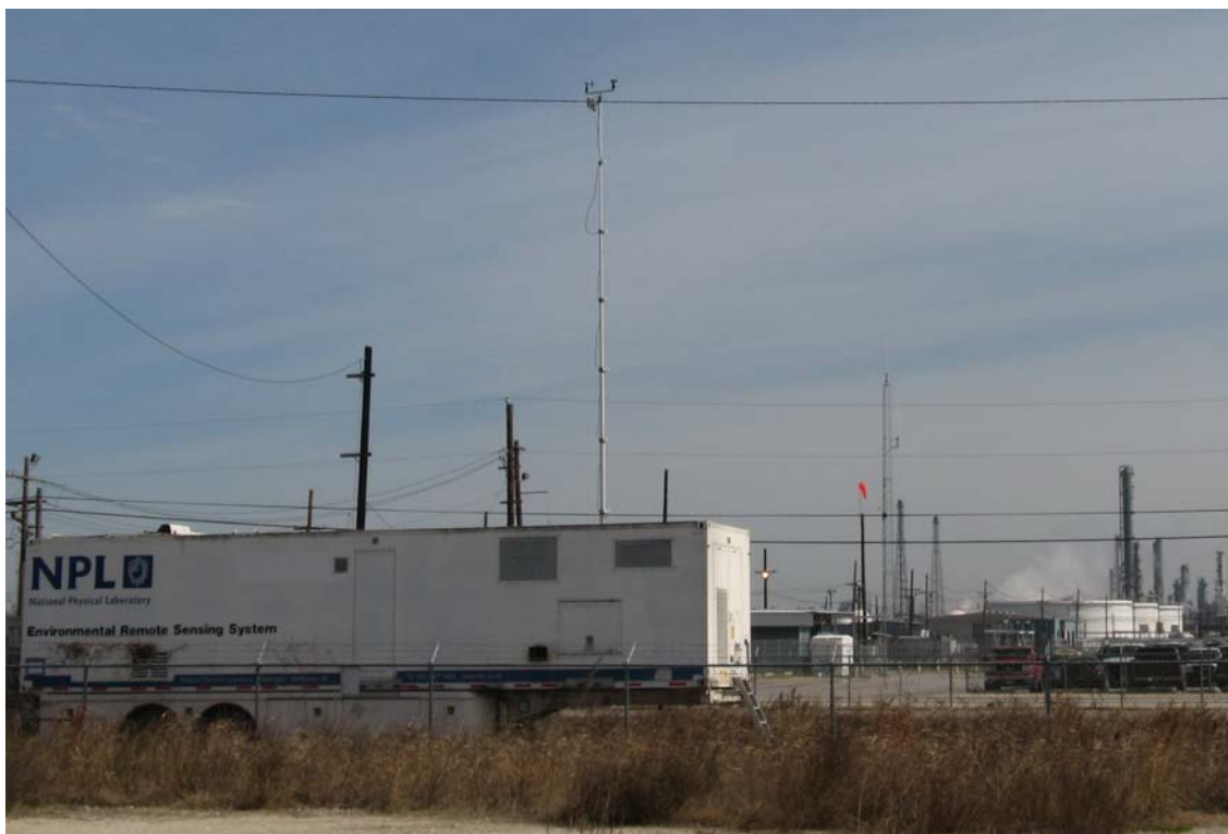
Figure 1.1 NPL DIAL facility on the Shell Deer Park site in Houston.
