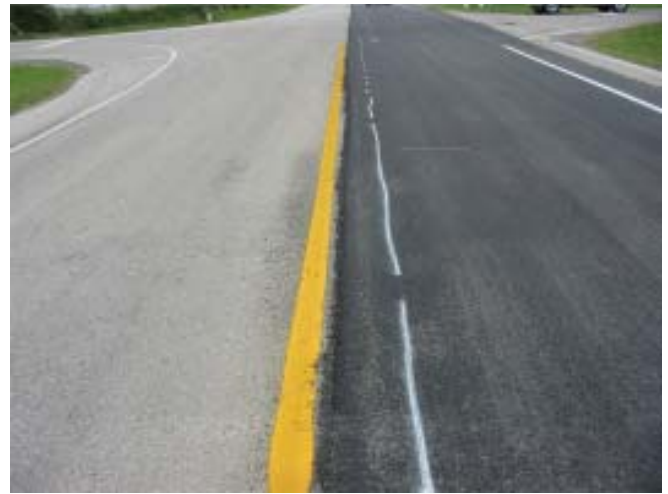
Aged (left) and new asphalt (right) in Hempstead, Texas. Photo courtesy of Dana Easley, 2003.
