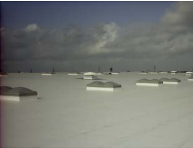
Reflective roofing installed on a University of Texas Health Science Center building in Houston.
