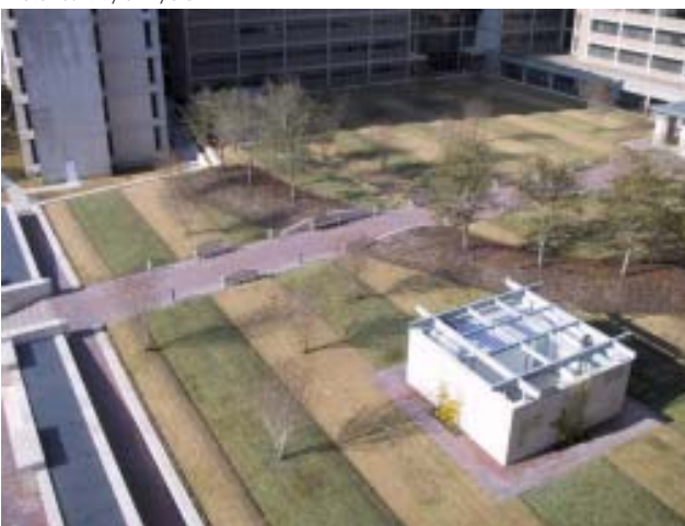
A green roof on the Baylor Research Institute in the Texas Medical Center provides intensive planting on top of this large structure.
