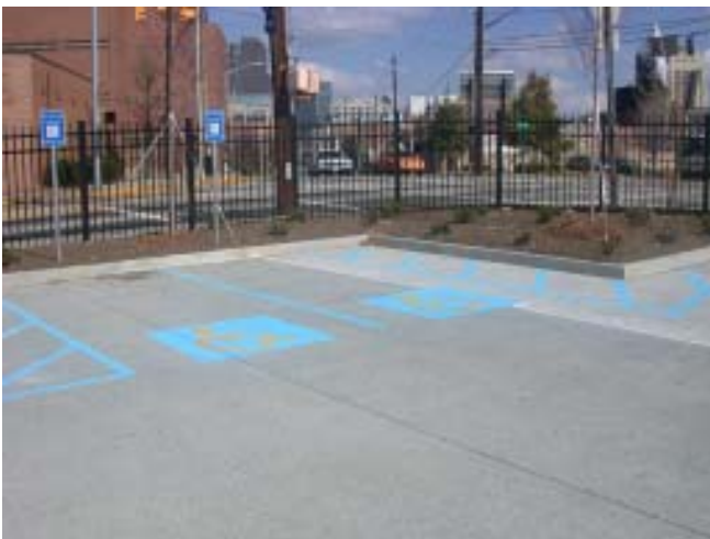
Example of porous concrete used on parking lot in Atlanta. Note that there are various porous concrete and paving options, available for a wide range of applications.
