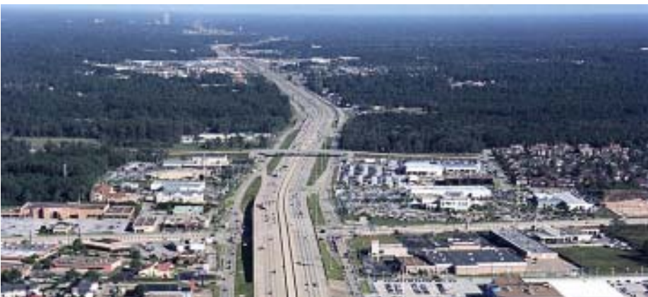
Urban development can involve removal of most of the existing tree canopy, as shown here on I-45 in a heavily forested area. Conservation measures are particularly important in such locations.
