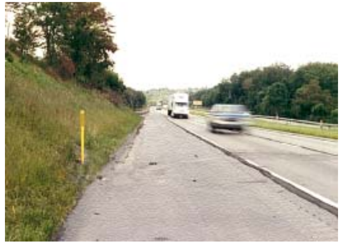
Porous paving and other cool paving products can be used for roadway shoulders to assist in runoff management while reducing the heat island affect.
