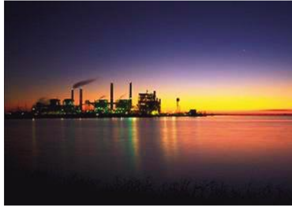
Texas Genco's W.A. Parish coal-fired power plant, a four-unit, 2,620-megawatt facility located in Fort Bend County, is among coal plants with the lowest NOx emissions in the nation. Photo courtesy of Texas Genco.
